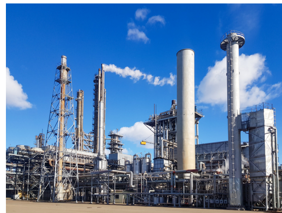
Petrochemical & Pharmaceutical Units
